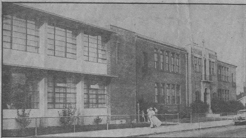
ST. MICHAEL'S TODAY —Golden jubilee year of St. Michael's School began with opening of modern four-classroom addition, left. Main school building, the third to be built, was completed in 1926. All former pupils have been invited to a reunion festival Oct. 18 at St. Michael's, 87th St. near Vermont. Charter pupils will be guests of honor.
